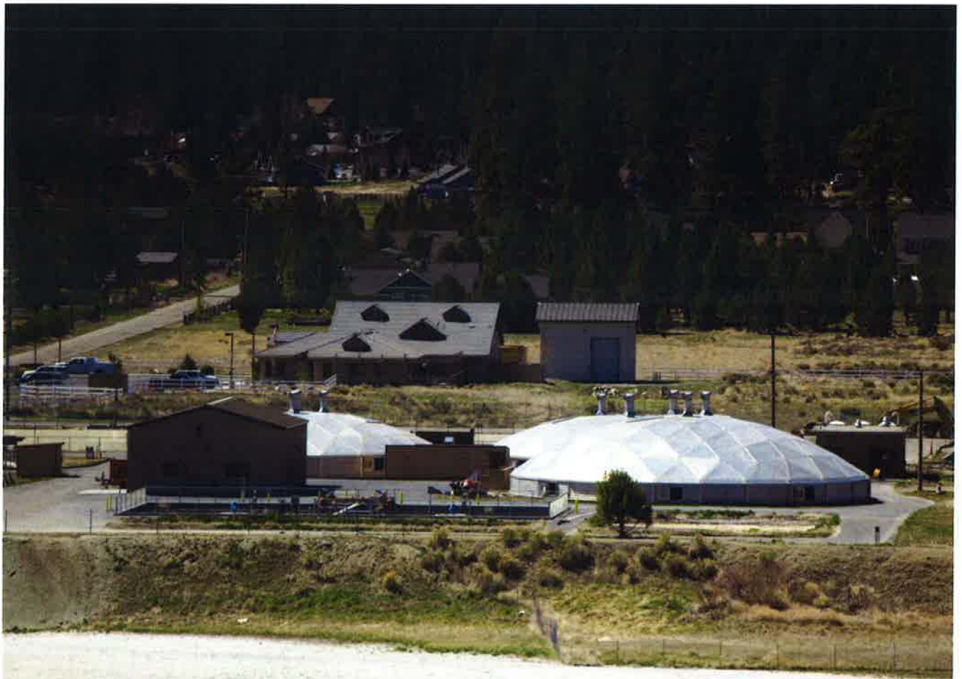
Treatment Plant, Big Bear City, CA
